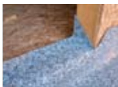
PRIOR TO INSTALL
